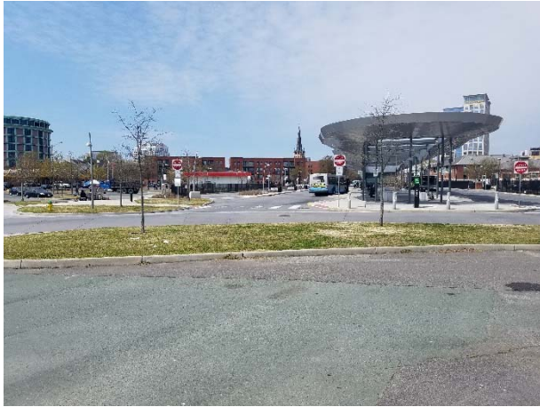
Photograph 37. View of the east side of the HRT bus terminal.
