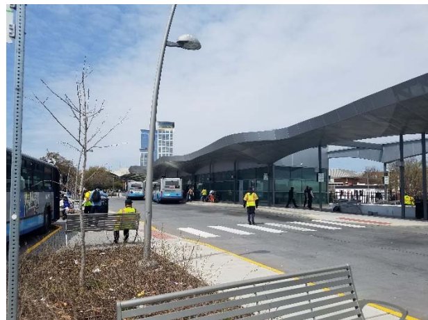
Photograph 40. View of the south side of the HRT bus terminal.
