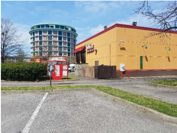
Photograph 4. View of the south side of the building and drive through.
