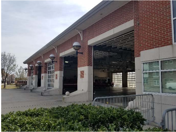
Photograph 49. View of the north side of the building and associated engine bays.
