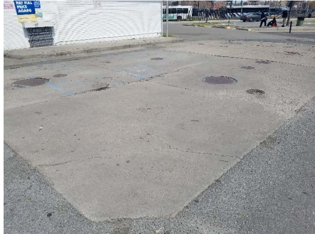
Photograph 26. View of the UST area.
