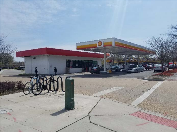
Photograph 22. View of the north and west sides of the building and associated fueling pump canopy.
