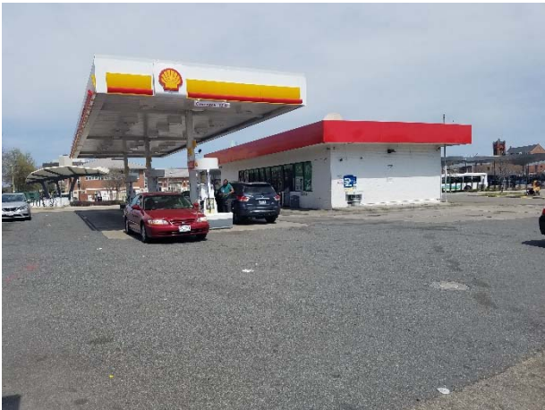
Photograph 23. View of the south side of the building and associated fueling pump canopy.
