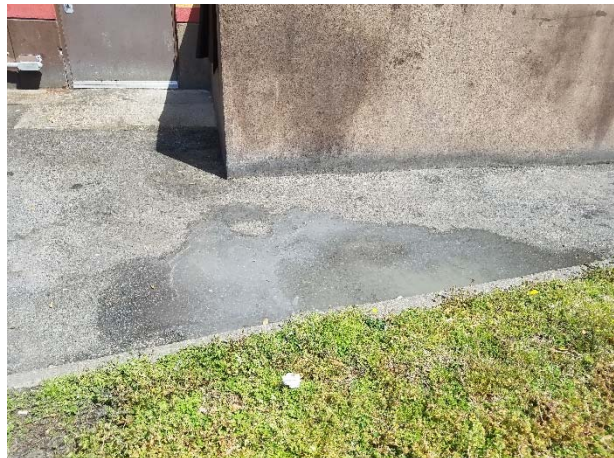
Photograph 8. View of the milky-white liquid substance pooled between the grease trap and storage shed.
