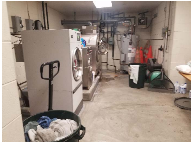
Photograph 60. View of the on-site laundry room and water heater.
