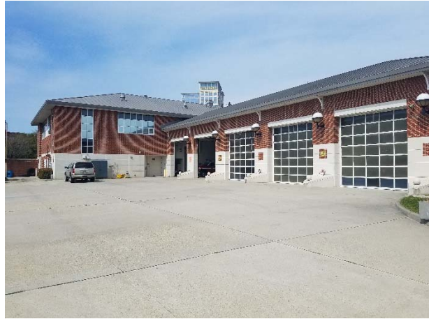
Photograph 50. View of the south side of the building and garage bays.
