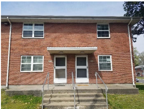
Photograph 75. View of two of the six units within a building.
