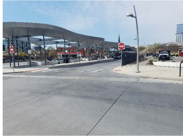
Photograph 38. View of the north side of the HRT bus terminal.
