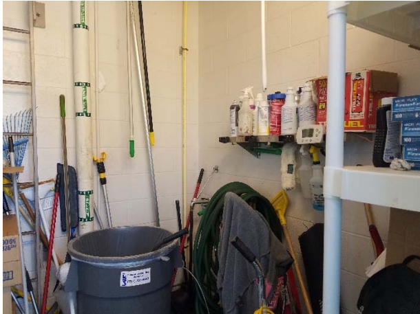
Photograph 47. View of the utility closet within the HRT bus terminal.
