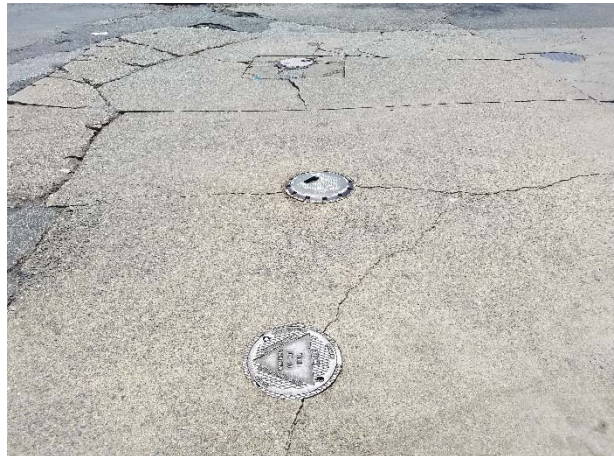
Photograph 28. View of the UST fill caps.
