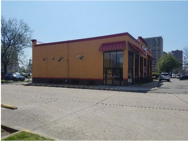
Photograph 2. View of the north side of the building.
