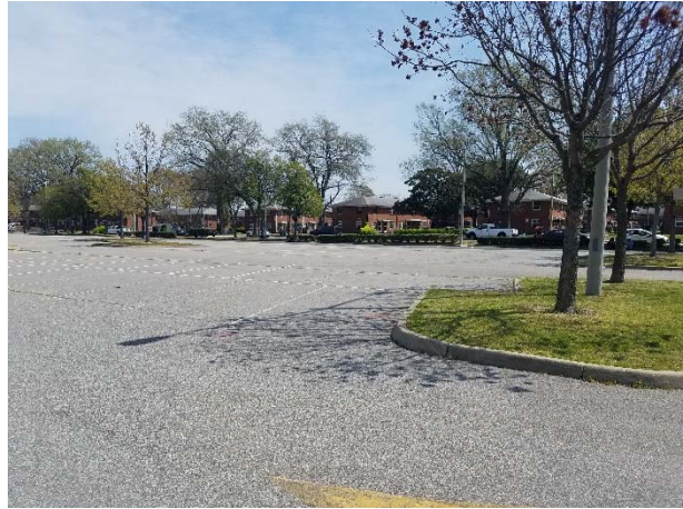
Photograph 74. View of the northern building units within the subject Site boundaries.
