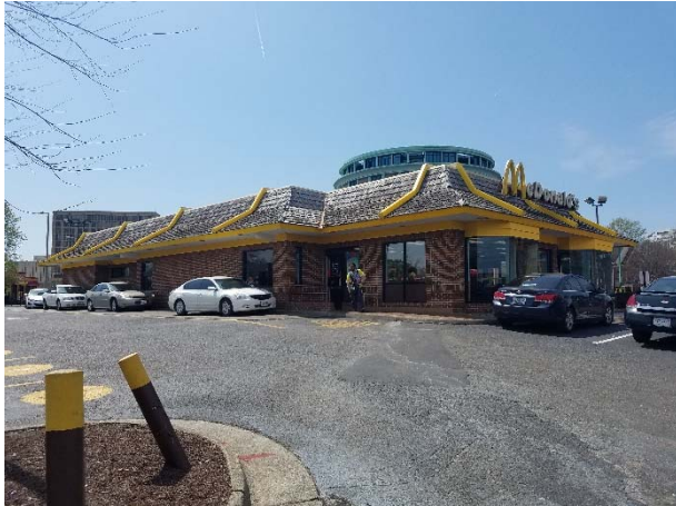
Photograph 17. View of the east and north sides of the building.
