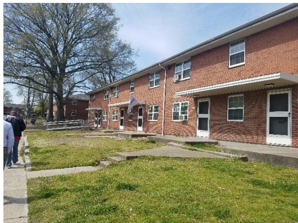
Photograph 76. View of the exterior of the building.
