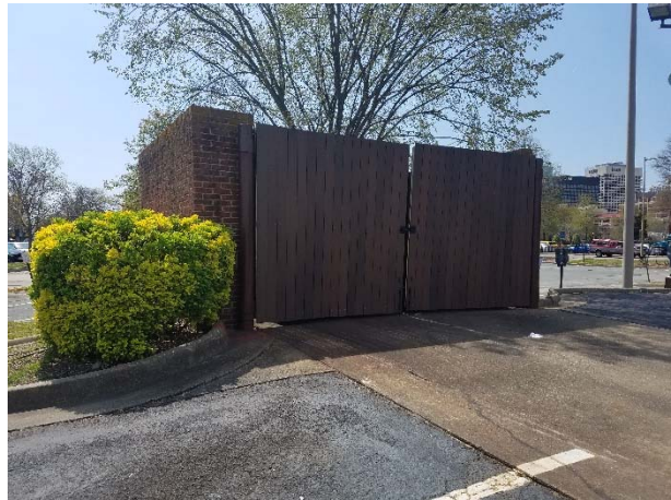
Photograph 20. View of the gated dumpster located on the south side of the property.
